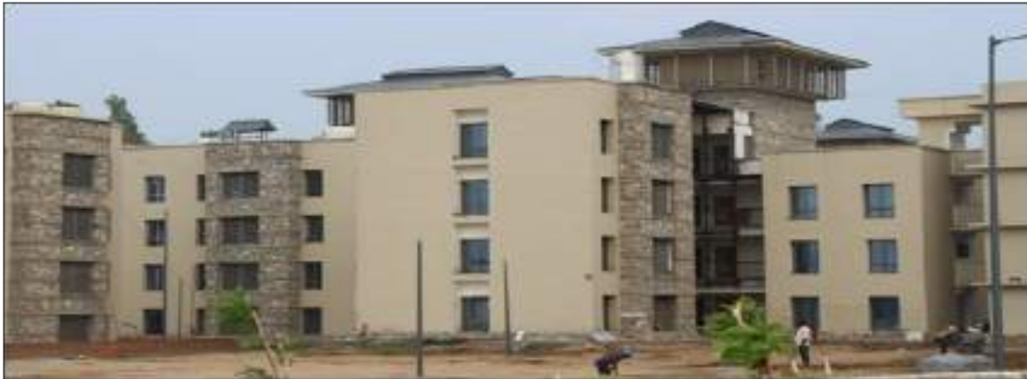
One of the hostel buildings at the permanent campus
